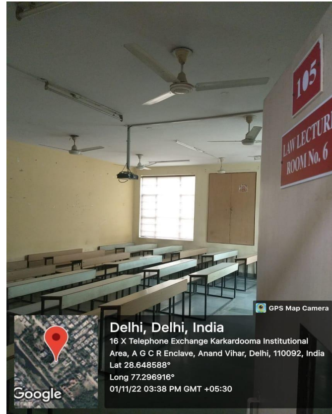
ROOM NO 105,WALL MOUNTED PROJECTOR
