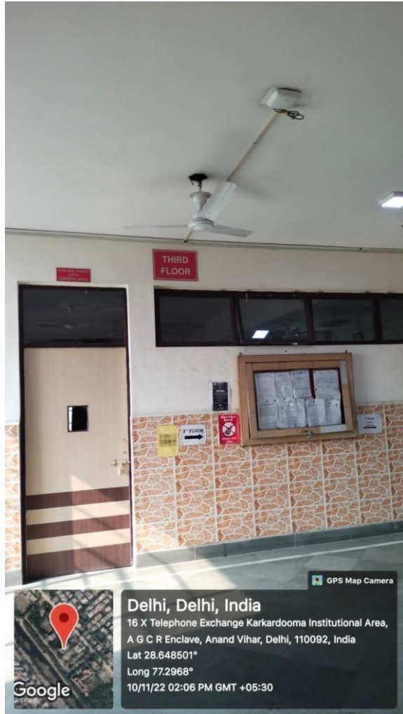
Third Floor, Wi-Fi Facility
