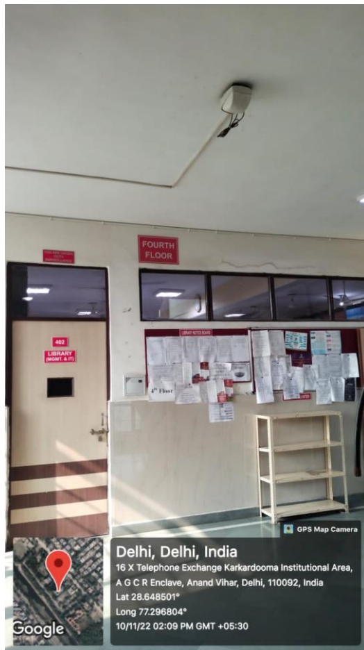
Fourth Floor, Wi-Fi Facility
